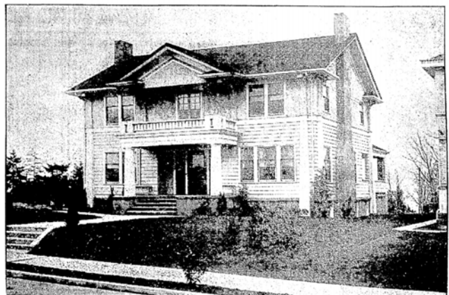
This fine big 9-room house, beautifully situated on a 60x135-foot lot, running through from street to street, is an exceptional offering on special terms. Living room and den are finished in Philippine mahogany with oak floors. Fireplaces in both den and living room. Hot water heat. Storage in basement with entrance from the rear. Shown by appointment.
